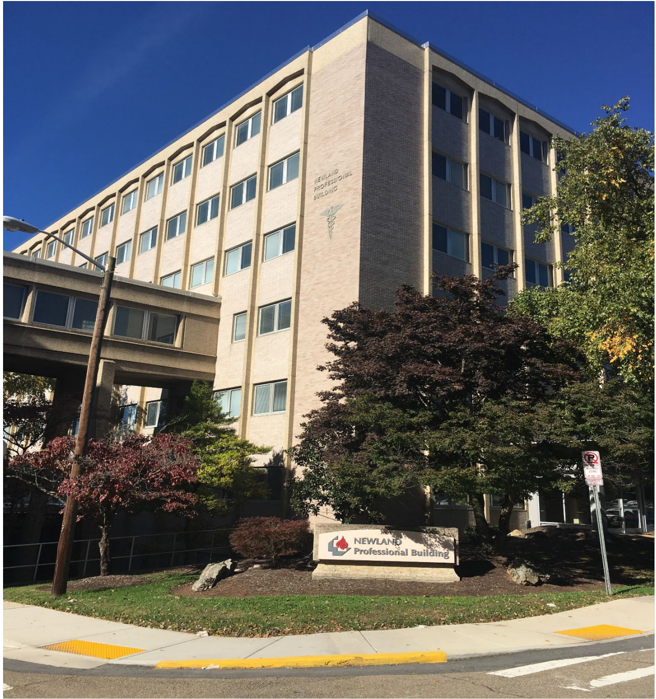
The Newland Professional Building, located at 2001 Laurel Avenue, Suites N-601, N-602, N-603, and N-604, Knoxville, TN 37916 is the location of the TWU MOT Program.
